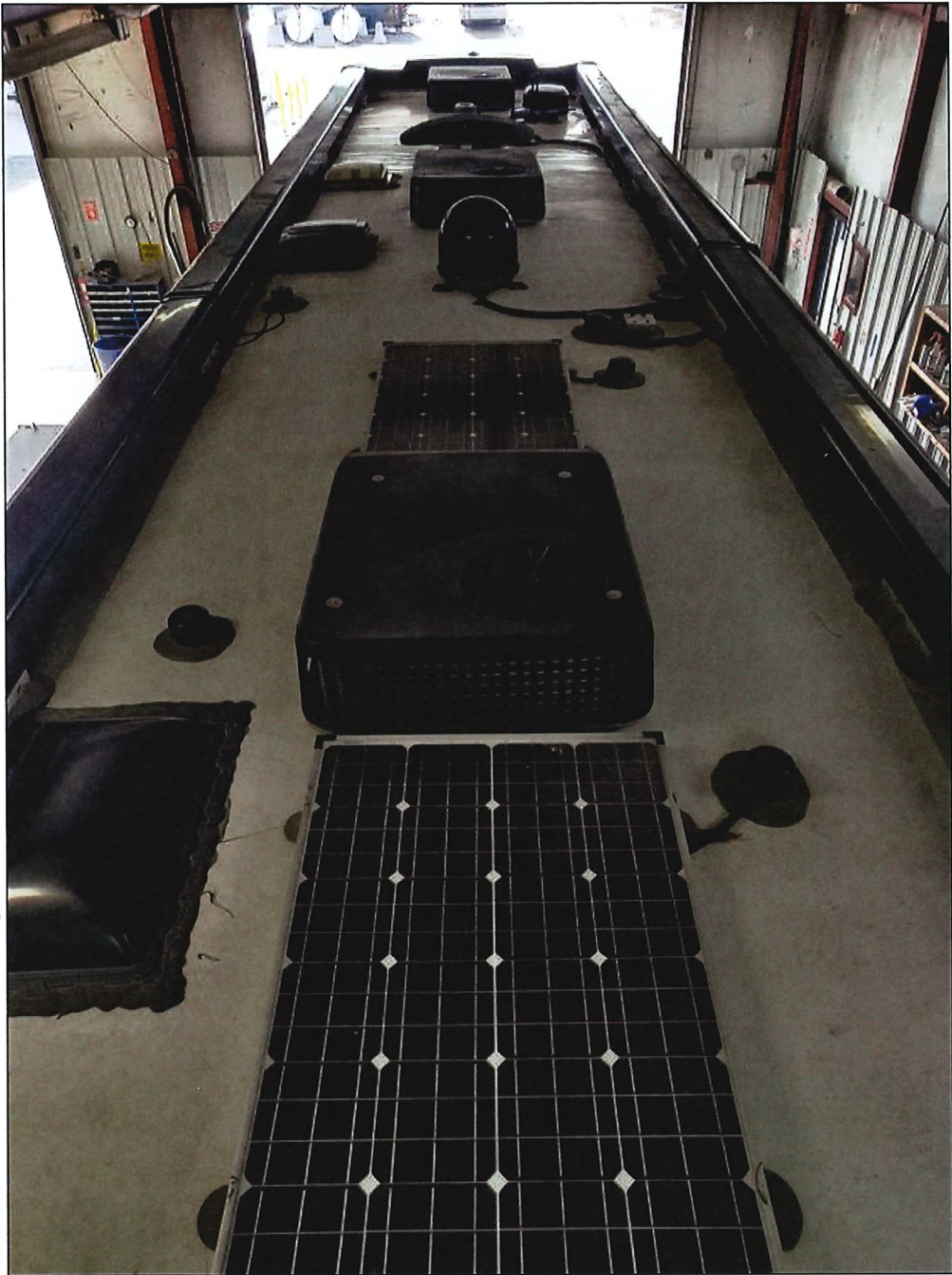
Roof Rear to Front
